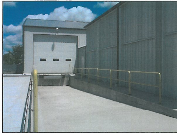
60'x18' Concrete Loading Dock
